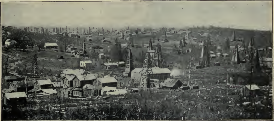
FIG. 161. — A view in the oil fields of western Pennsylvania. Each of these small towers, or derricks, stands over an oil well. The derricks were used in boring the wells.
